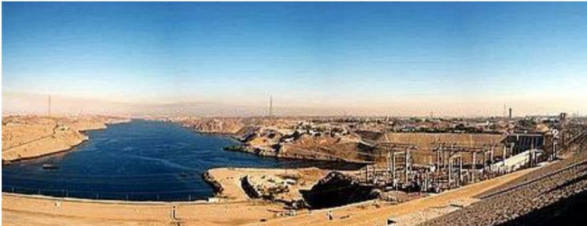
Aswan Dam – Egypt
